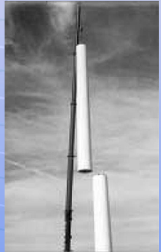
Installation of Tubular Tower
