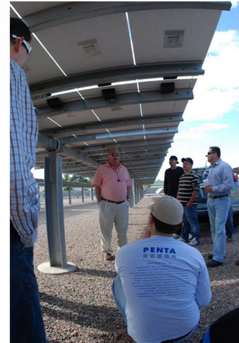
15 year old 200KW SRP Power plant Tempe AZ
