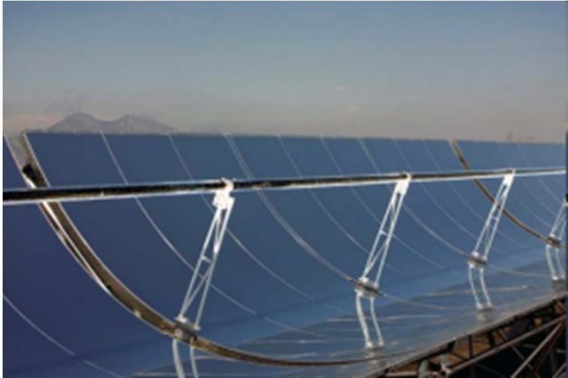
Large arrays of mirror troughs heat a working fluid to very high temperatures
