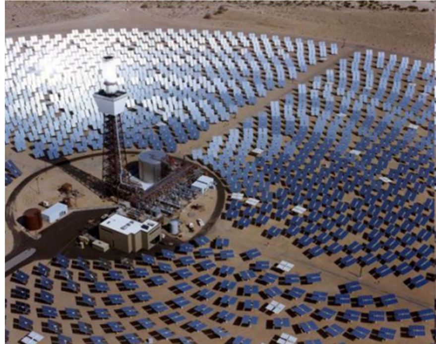
Large sets of Heliostats can work together as a lens and reflector
