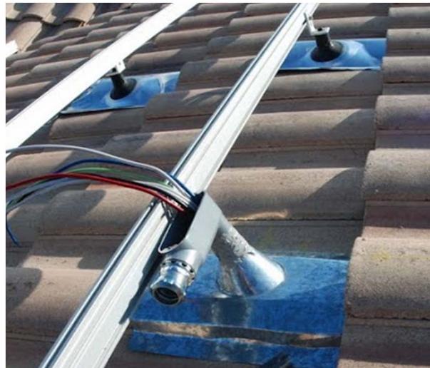
Array, sensors, support equipment, rails and standoffs with flashing, tie into grid via breaker
