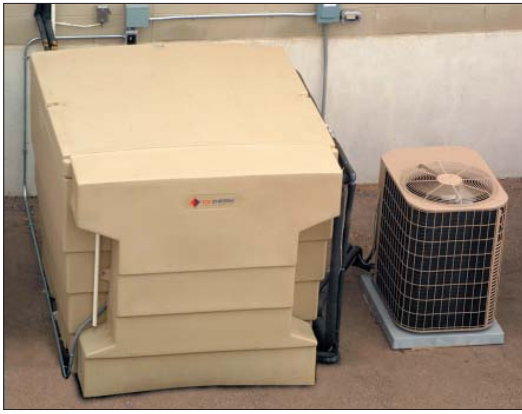
Ice Energy's Ice Bear energy storage system can reduce a building's cooling-related peak demand charges by 95%.
