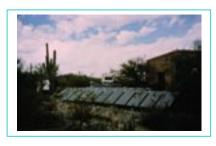
Rural Arizona application of this strategy has been applied to passive water heating (thermosiphon), or for radiant floors. Since hot water rises, and cold water settles, the thermosiphon system has the collector lower than the tank or application. This convective loop runs continuously as the sun shines
