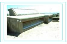
This solar/day lighting element can also include operable windows and glazing to facilitate building natural ventilation exhaust of unwanted interior heat. Now there are four functions for one building element. It provides natural illumination; it provides for natural ventilation and building cooling; it provides a place for solar water or photovoltaic panels, and it provides an interesting and dramatic building design element
